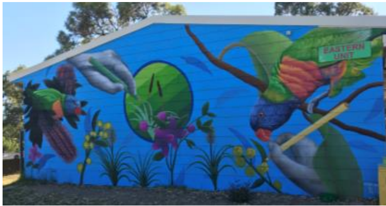
The Eastern Unit houses teaching areas Spanish and Performing Arts
